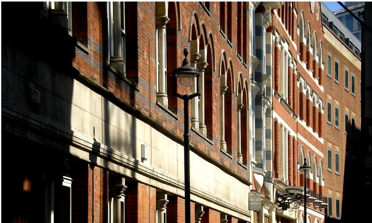
Breams Buildings, North side (detail0
